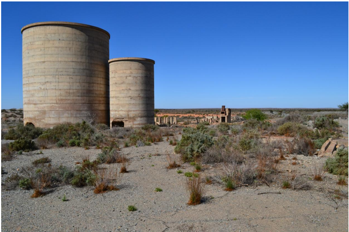
Ore storage bins at the Radium Hill mine site (B.Chandler photo)
